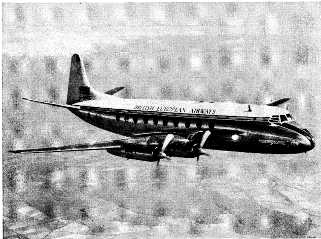
Vickers Viscount, 1948. The first turboprop airliner, this British model used by U.S. lines carries up to 48 passengers at 315 m.p.h. for 1,400 mi.
