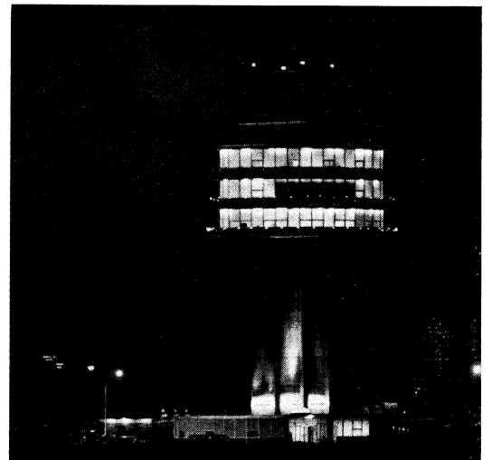
Newark, N.J., airport control tower at night. The 150-ft. tower, located between the two active runways, is electronically equipped to guide air and ground aircraft traffic
