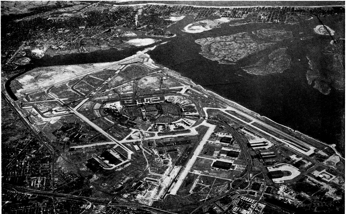
New York International airport (Idlewild), Queens. Under construction since 1942, it has facilities for accommodating all types of aircraft traffic, ranging from local commuter helicopters to long-distance transcontinental jet planes
