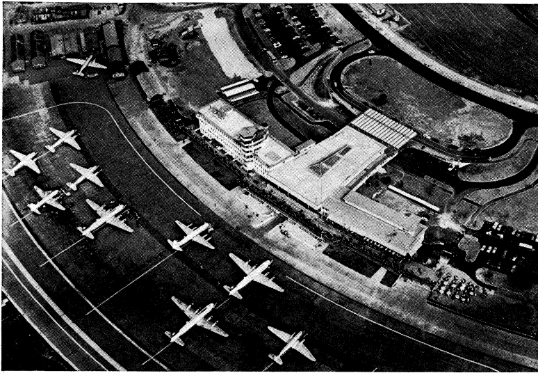
Zürich airport at Kloten, Switz., 7½ mi. from Zürich, showing the terminal building, with built-in control tower, and the passenger loading area
