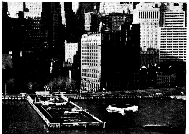
New York downtown heliport on the East river, showing the 80- by 85-ft. landing strip. Manhattan's second heliport, put into operation in 1960, it provided 22 daily flights to and from LaGuardia, Idlewild and Newark (N.J.) airports
